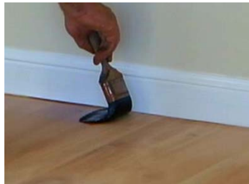
Cutting in the finish around perimeter walls.
