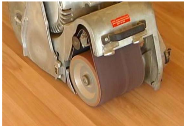
Third pass of sanding in the board direction.
