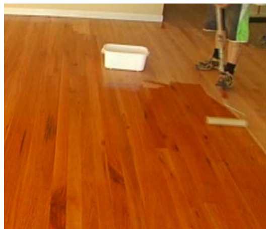
Application of the initial coat.
