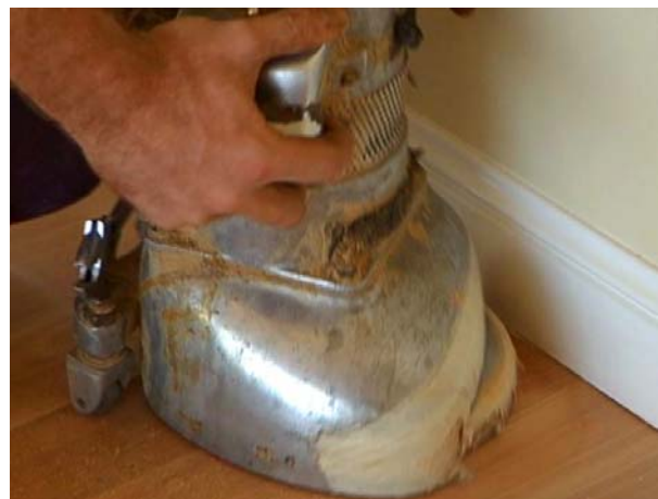
Edge sanding require a smooth action to blend into the floor.
