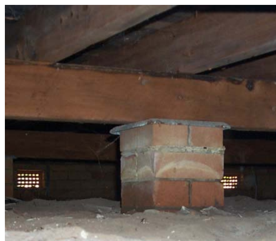
A dry sub-floor space and adequate ventilation is essential for floor performance.
