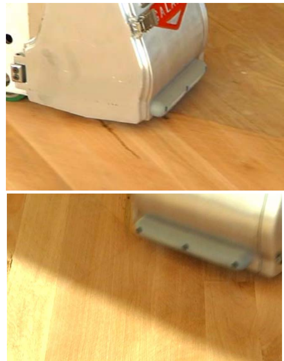
First and second pass of sanding at 45° to board direction.
