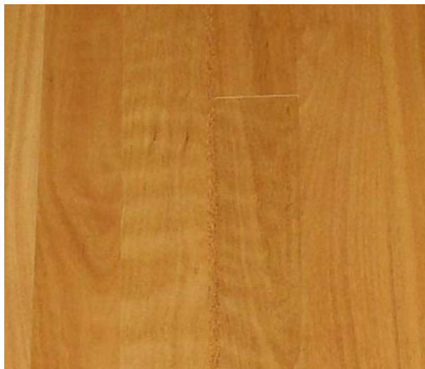
Cork intermediate expansion joints blend in well with timber floors.
