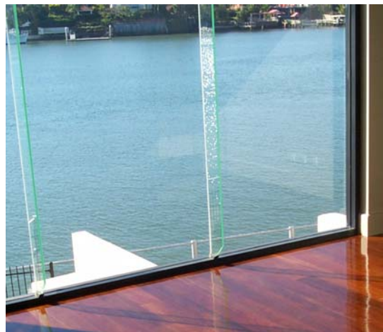
Greater localized shrinkage and possibly some cupping can be expected with high sun exposure.
